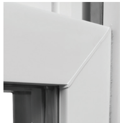
Fusion-welded corners prevent air from passing through and boost structural support.
